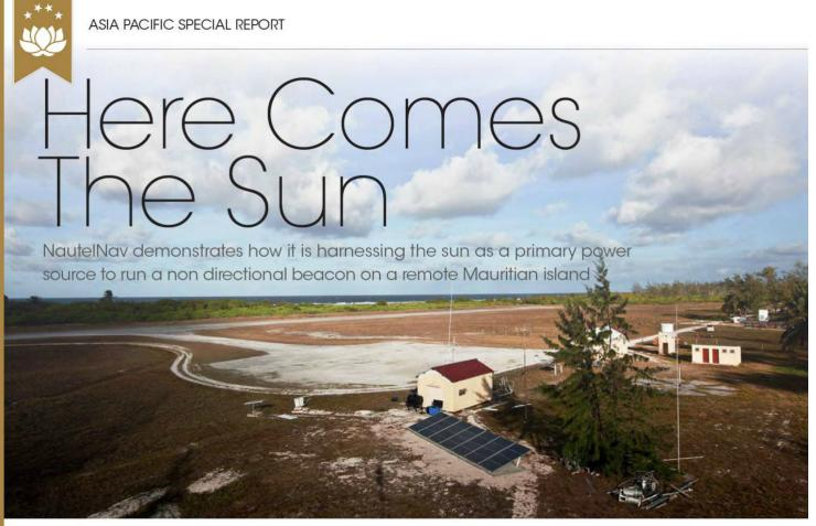
on directional beacons (NDB) are often located in extremely remote sites, and many do not have readily available AC power. And while some may have AC power, it can be unreliable. Rather than exclusively using generators, which can be costly and maintenance-intensive, some municipalities are opting to use solar power as the primary power source with generators as backup.
